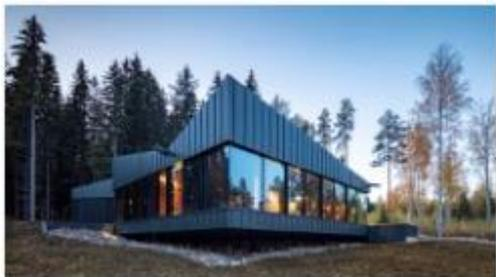
Just as the colour of the dark wood lathing on the façade is oriented to the surroundings, the dark shimmering RHEINZINK titanium zinc elements blend in just as appropriately.
