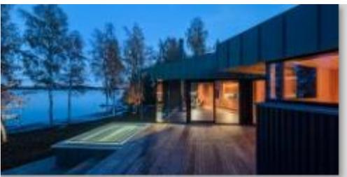
The surfaces above and below this horizontal façade coil are panelling with RHEINZINK titanium zinc in RHEINZINK-prePATINA graphite-grey surface finish.
