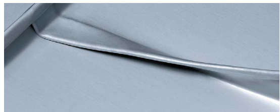
Rounded seam connection (1a) Upstand \geq 150 mm with water check, pinched seam round seamed to double standing seam
