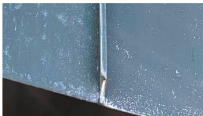
Examples of salt deposits on façades, seams and drip edges
