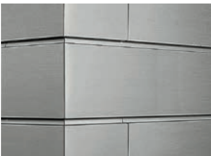
RHEINZINK-Panel H 25 with 20 mm joint and slave profile
