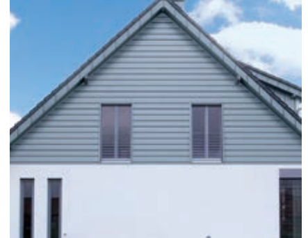
Gable cladding at residential building
