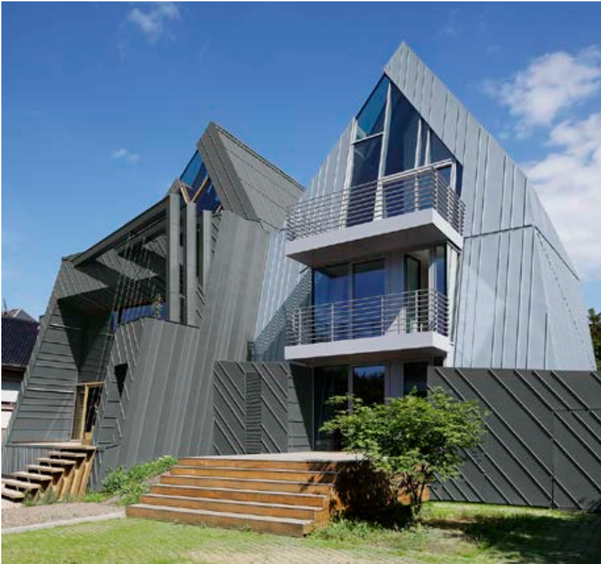
Residential and office building, Grevenmacher, Luxemburg
