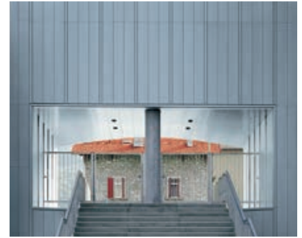
Telecom Giubiasco, Giubiasco, Switzerland
