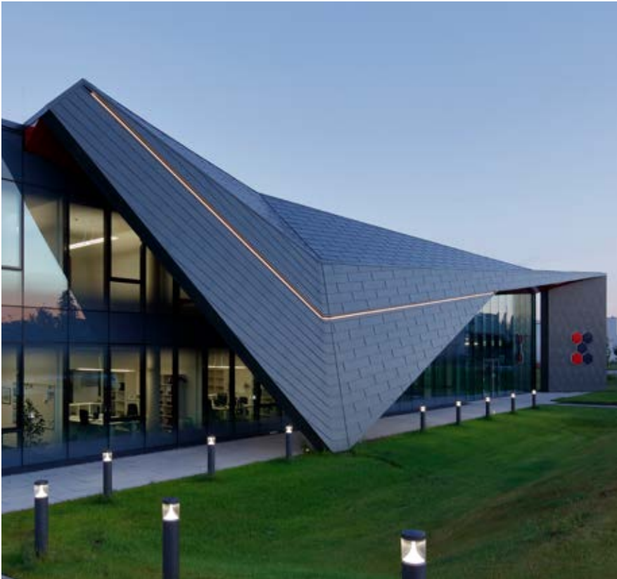
Office Building, Wedemark, Germany
