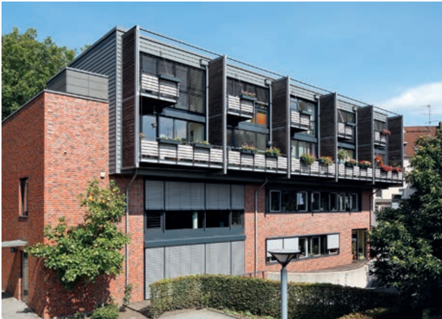
Residential Building Duisburg-Hamborn e. G., Duisburg, Germany
