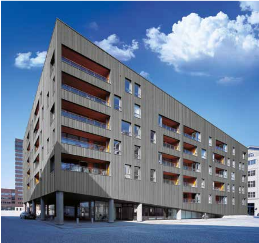
Zinkhaus, Copenhaga, Danemarca
